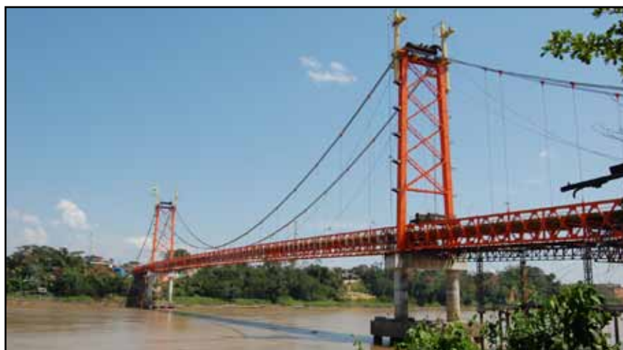
Figure 3: Trans-Oceanic Highway: bridge nearing completion in Puerto Maldonado
